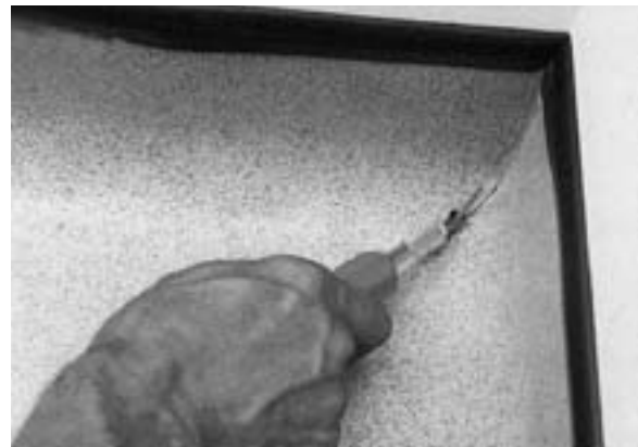
2. Trim the weldrod with the round router blade.
