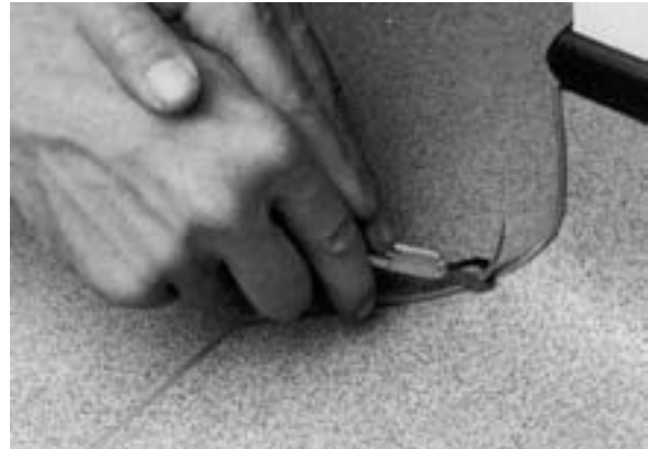
4. Chamfer off the external mitre with the square router blade.
